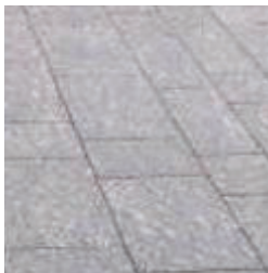
shared path & median_ milled concrete pavers
