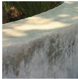
wall material_ formed concrete walls
