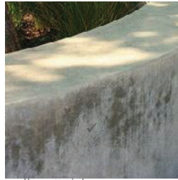
wall material_ formed concrete walls
