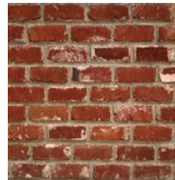
wall material_ recycled brick walls
