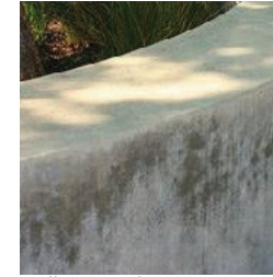
wall material_ formed concrete walls
