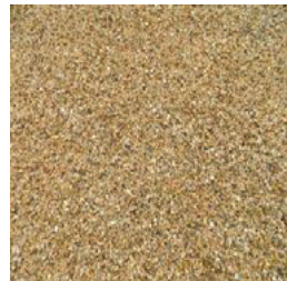
surface treatment_ stabilised gravel
