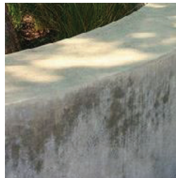
wall material_ formed concrete walls
