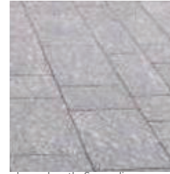
shared path & median_ milled concrete pavers
