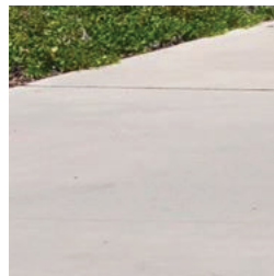
shared path_ brushed concrete
