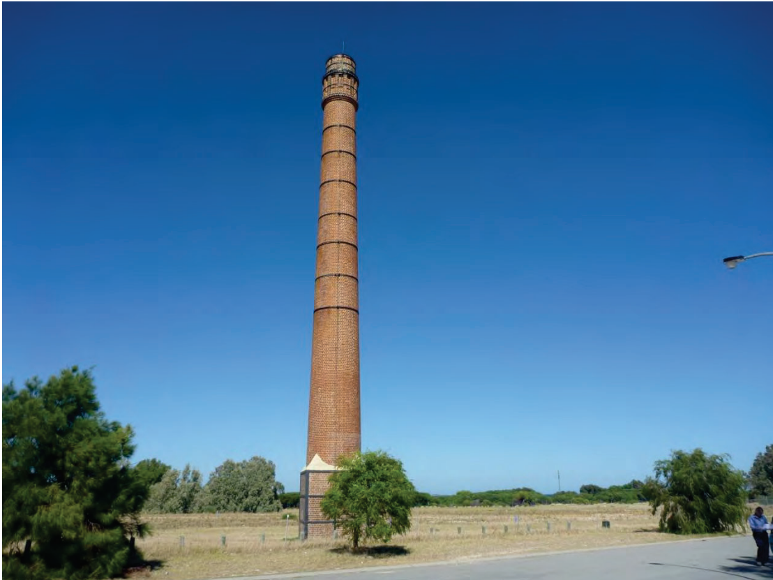
Plate 8 Robb Jetty Chimney (a Heritage listed place) is within the study site)
