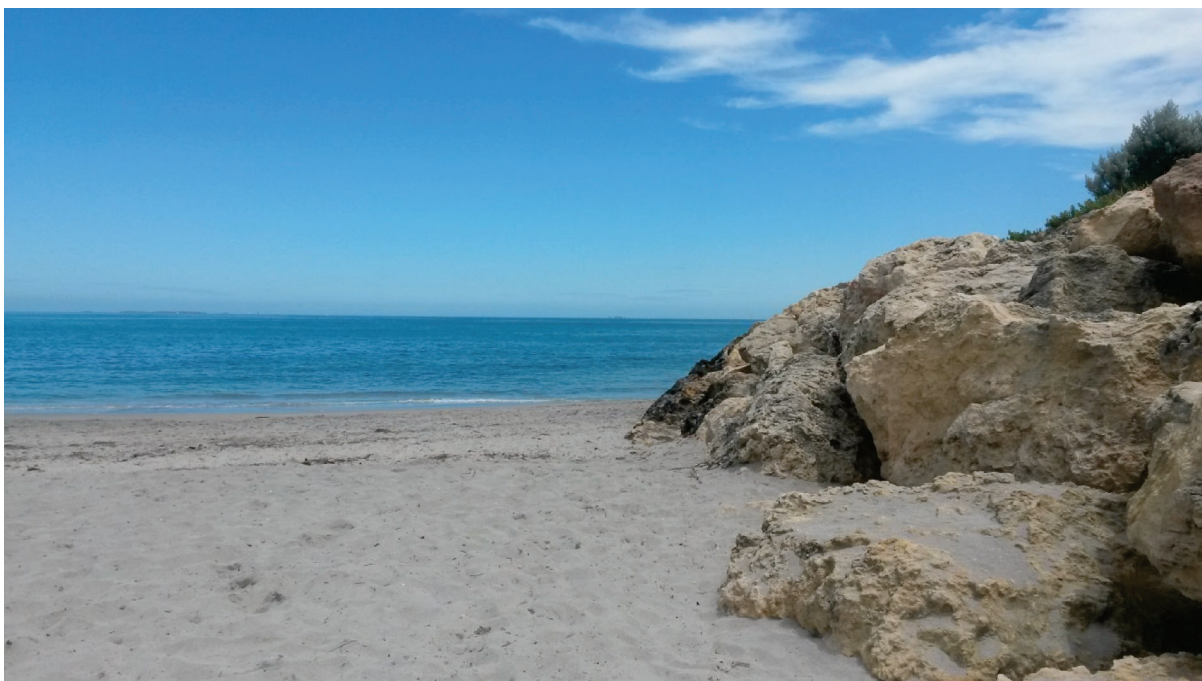
Existing interim protection (groyne) at the north of the City of Cockburn.
