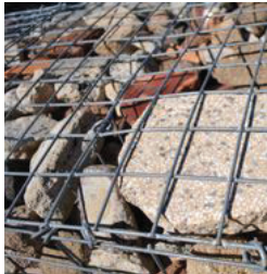
wall material_ gabion walls
