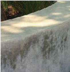
wall material_ formed concrete walls
