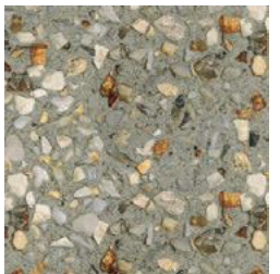
shared path_ washed aggregate concrete
